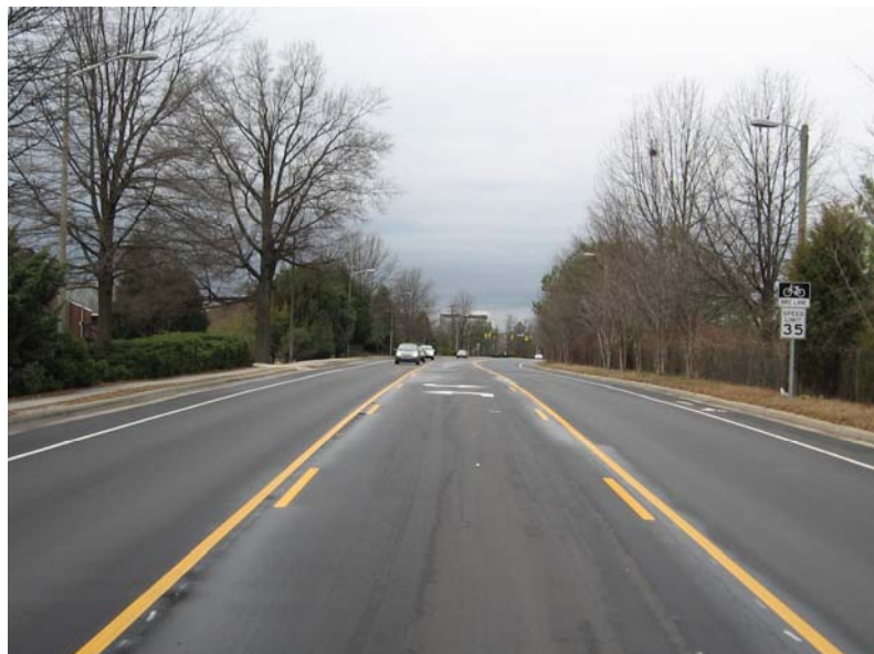
Erwin Road after restriping (three motor vehicle lanes with bike lanes).
