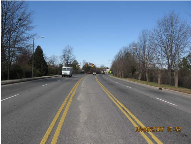
Erwin Road prior to restriping (four motor vehicle lanes).
